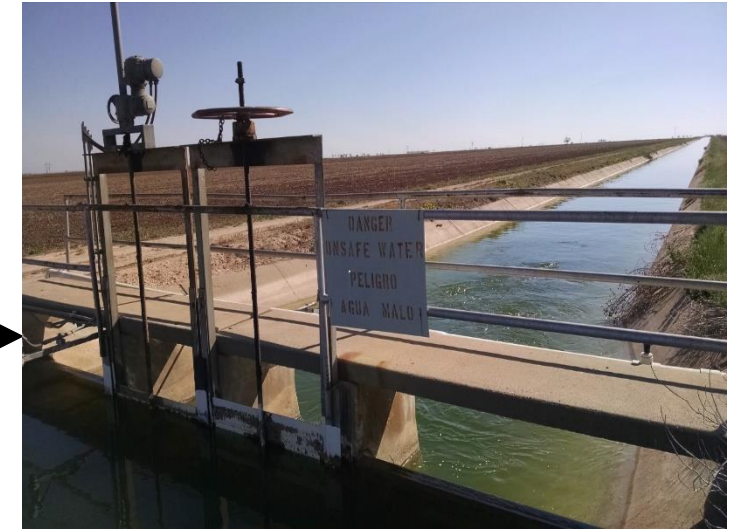
Treated Wastewater Source: Canal holding treated wastewater
